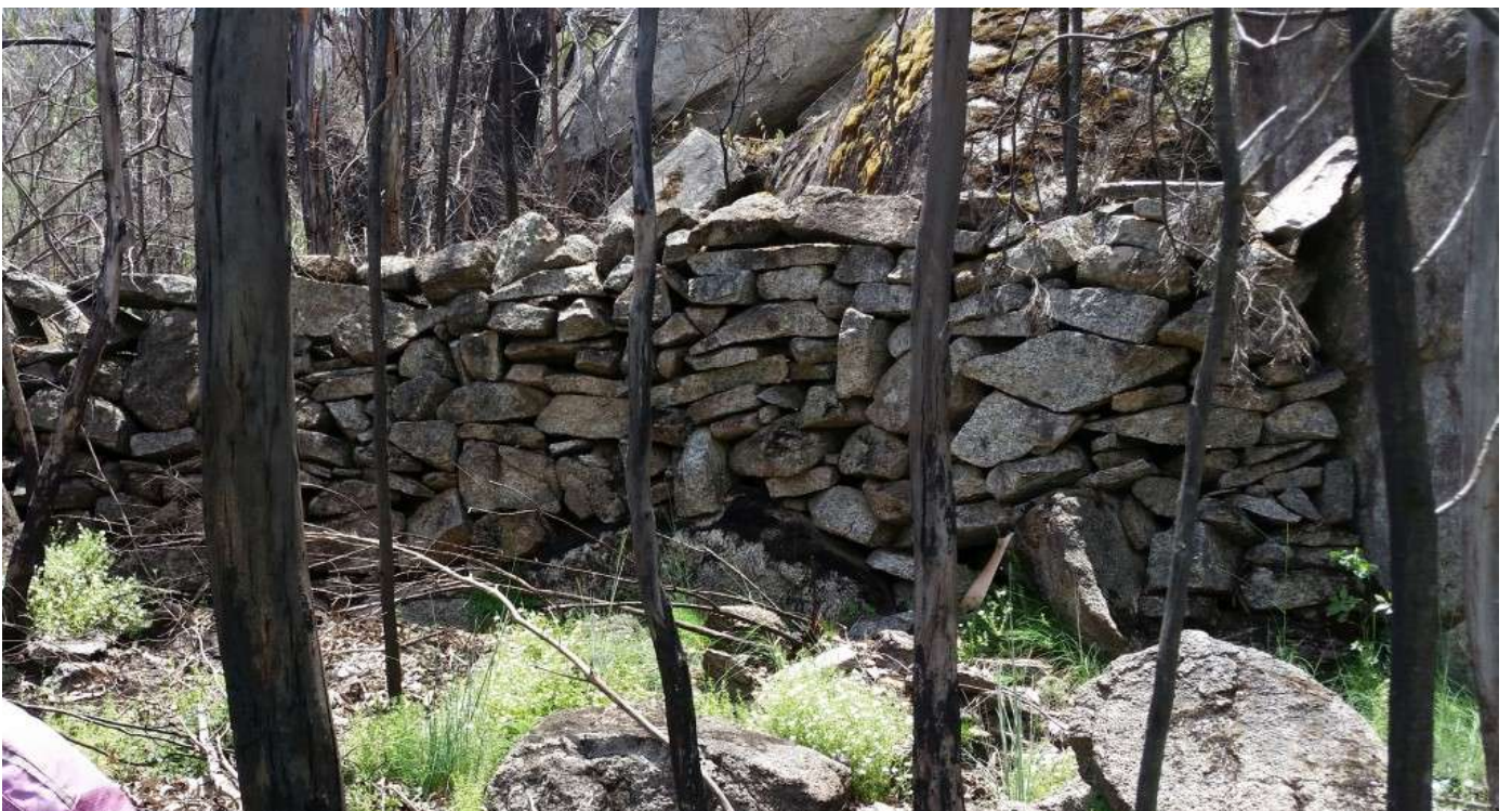
One of the old stone walls above Glendale Depot
