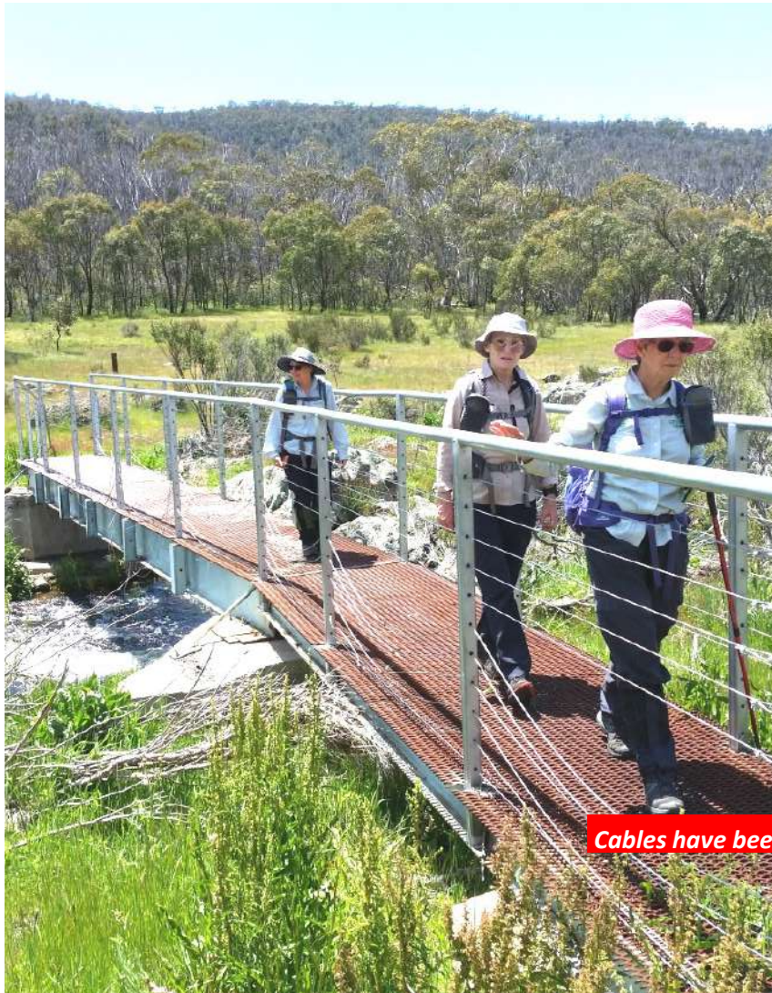
Heritage Trail bridge over Orroral River
