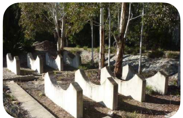
Foundations supporting diesel fuel tanks at the Tracking Station
