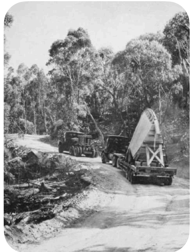
The counterweight for Honeysuckle's 26 metre antenna being taken up the steep and winding old Apollo Road.
