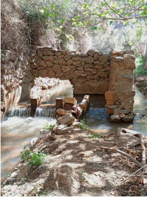
The old irrigation systems still work well
