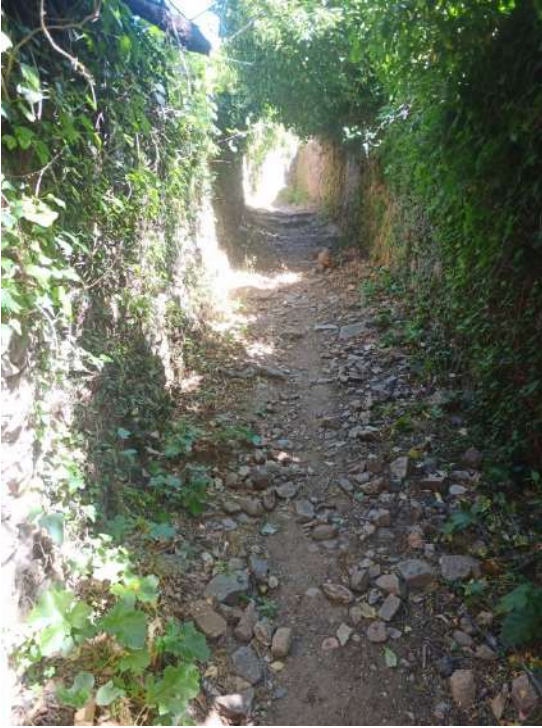
Stone walls each side of the track
